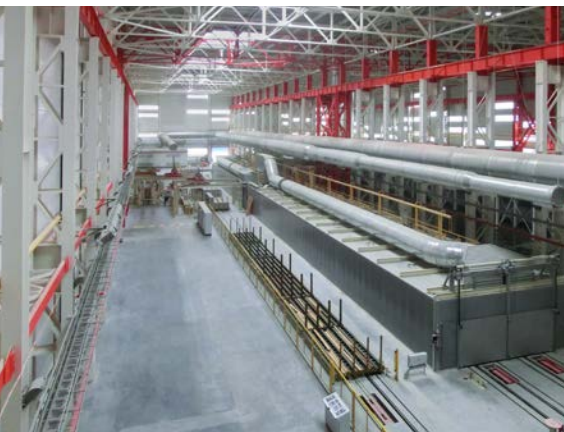
Grenzbach gypsum block dryer, view from the inlet side
