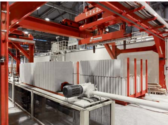
Gypsum block unloading and compacting unit
